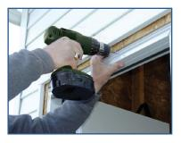
4. Screw jamb covers to the jambs. 5. Snap on the new brickmould.
