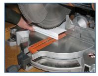
3. Cut jamb cover & brickmould.
