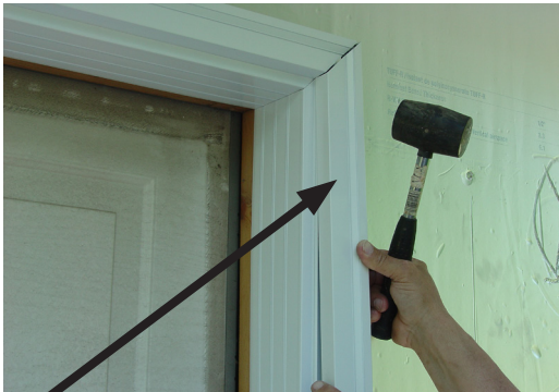
The brickmould casing snaps onto the locking legs on the jamb cover.
