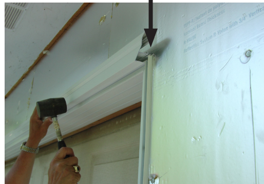
The brickmould casing snaps onto the locking legs on the jamb cover.
