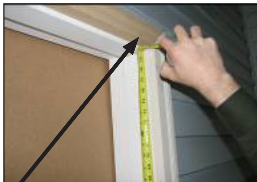
Measure from the inside of the header down to the sill.
