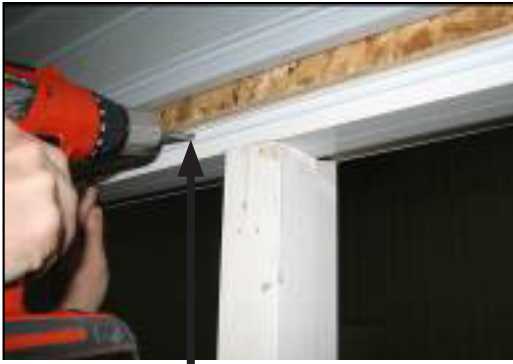
Install screws between the two locking points on the jamb cover.
