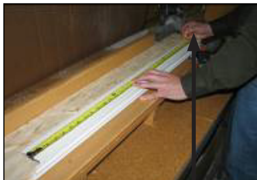
Transfer the dimension to the mull post cover for the proper length cut.
