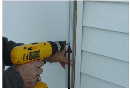
Screw to door jamb between the jamb cover locking points with pan head screws.
