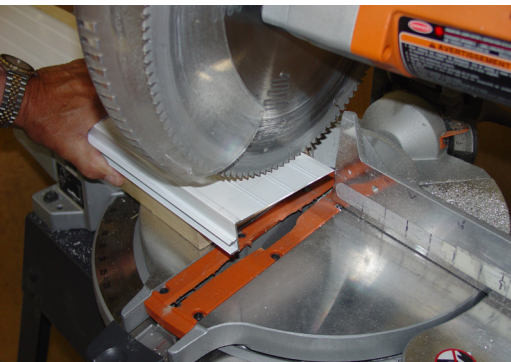
Transfer the side dimension to the aluminum side jamb cover.
