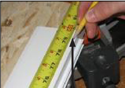
Transfer the side dimension to the aluminum side jamb cover.
