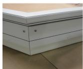
Assembled corners should have minimum separation between aluminum header and vertical jamb along the exposed jamb face and nosing.
