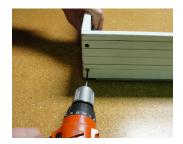
STEP 2: Attach the sill to the vertical jamb using screws or staples.
