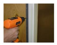
**STEP 12:** Using wood shims (not provided), shim until plumb and square vertical fame legs and arch top header, and fasten with screws or nails (not provided) through exposed nailing strip on frame verticals and arch top header.
