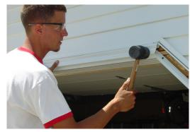
**Note**: Tap the casing onto the locking points with a rubber mallet.
