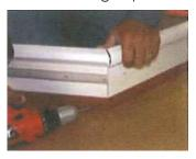
Assembled corner should have minimum separation between arch top and vertical leg along the exposed aluminum jamb face and nosing.
