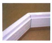
**STEP 7:** Using screw gun, on the backside of the vertical fame leg, through frame nailing strip, insert 3" drywall screw joining vertical leg nailing strip with header nailing strip as shown.
