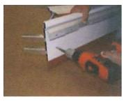
**STEP 6:** Insert mitered end of all-aluminum vertical frame leg into mating arch top header gusset(s). Gussets are designed to bend in center to allow arch top header and vertical leg miter to form clean tight mitered corner.
