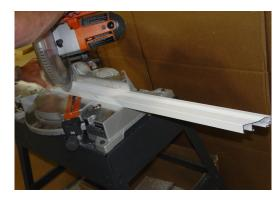
Note: Make sure the miters at the top are tight. If the miters are not tight, tap the brickmould up from the bottom and it will slide the brickmould on the jamb cover to create a tight miter
