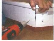
**STEP 9:** Using screw gun, insert one (1) # 6 x 2" PH screw from backside of vertical fame leg into leg of each inserted gusset.
