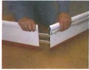
Assembled corner should have minimum separation between arch top and vertical leg along the exposed aluminum jamb face and nosing.
