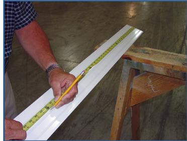
2. Measure door jamb & transfer dimensions to cladding.
